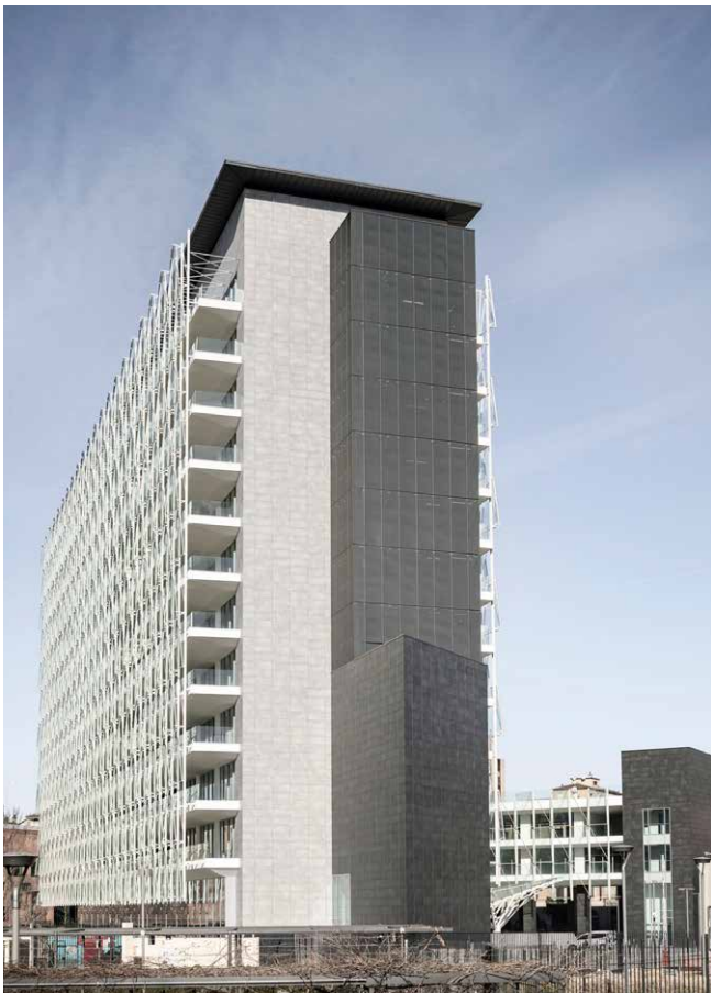
External facade, floors and columns Fiandre Core Shade Active in Cloudy and Sharp De Castillia 23 by Progetto CMR
