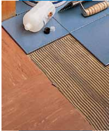
Laying on an old PVC floor
